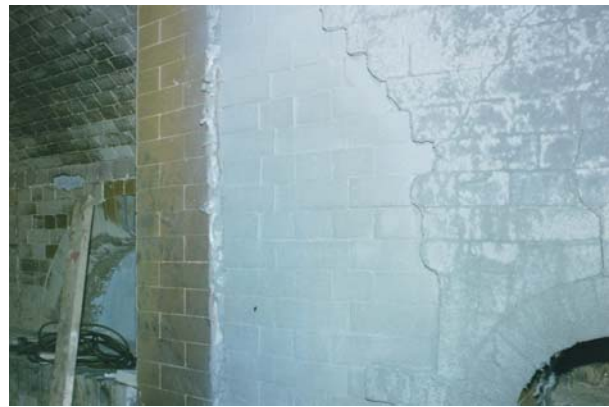
Fig. 7: Tunnel kiln preheat section (right 2/3 of photo) after application of high emissivity coating. The textural differences between the new and used refractory brick surfaces are obvious.
